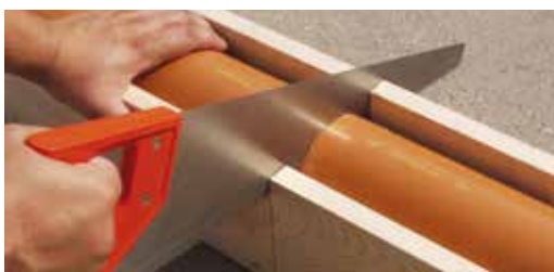
Figure 2 Pipe cutting with a hand-saw
