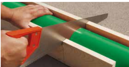
Figure 10 Shortening a Pipe with a Saw
