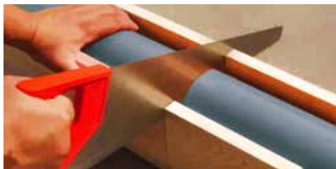
Figure 1 Pipe cutting with a hand-saw
